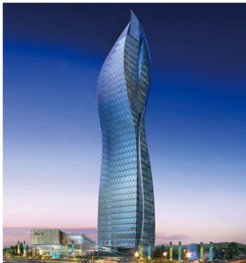
Tháp SOCAR, Azerbaijan SOCAR Tower, Azerbaijan
